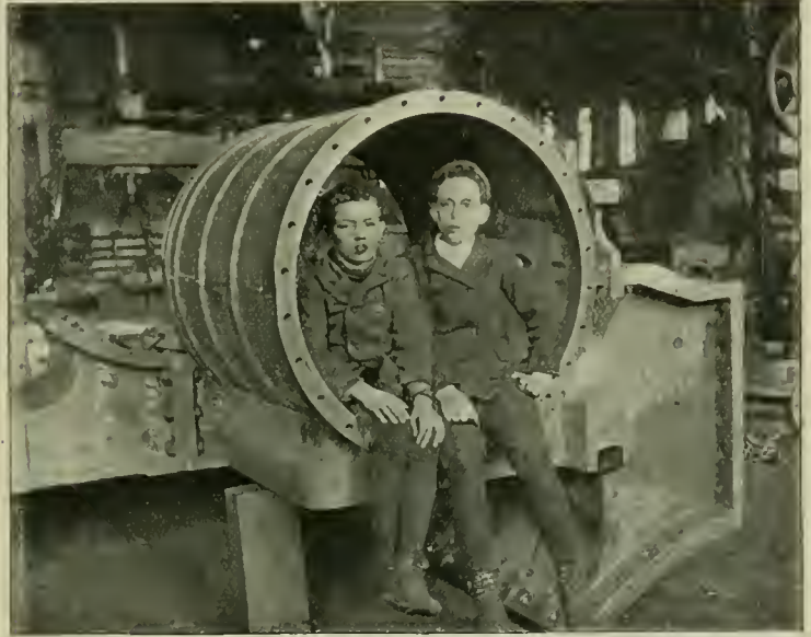
LOW PRESSURE CYLINDER, BALDWIN TWO-CYLINDER COMPOUND.
